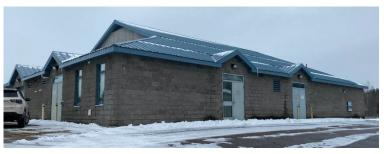
provides full conventional treatment to raw water drawn from the South River. The water treatment facility consists of two (2) Conventional Napier Reid package plants. An in ground clear well reservoir located under the facility has the approximate capacity of 1,536 m³ of useable storage. High lift pumps at the treatment facility run continually to maintain water pressure in the water distribution system piping.
